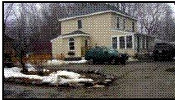
RESIDENTIAL HOME - BAR HARBOR, ME Complete rewiring as part of a major renovation.
