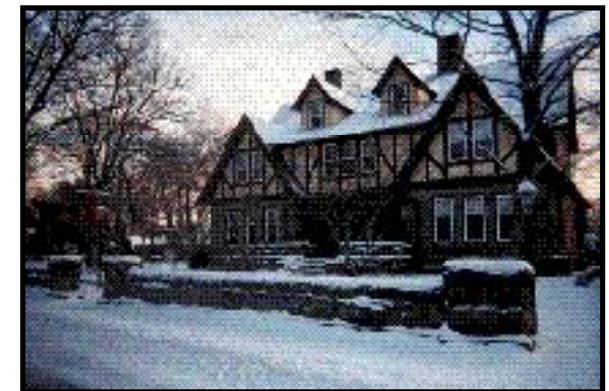
ATLANTEAN INN - BAR HARBOR, ME Complete interior electrical system upgrade.
